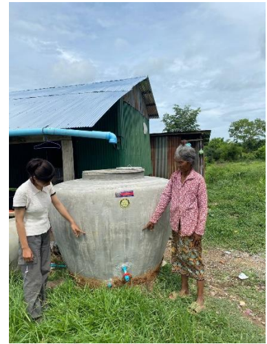
Roof changed, remove broken jar and replace big one
