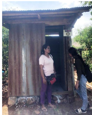
Latrine completely built and usable
