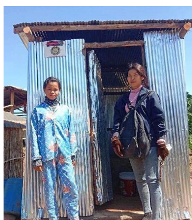
Latrine completely built and usable
