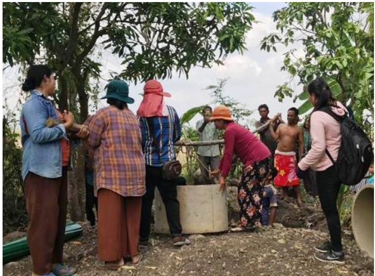
(Villagers help each other to build their latrines)
