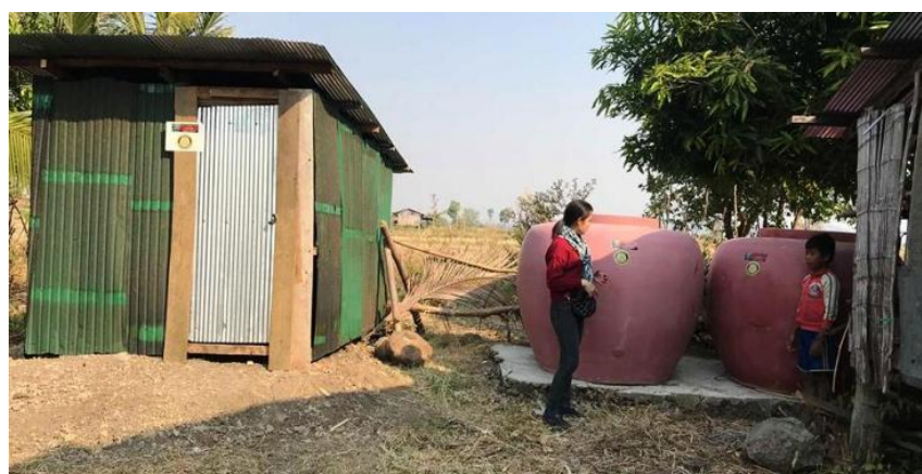
(Latrines and jars provided by CFS)
