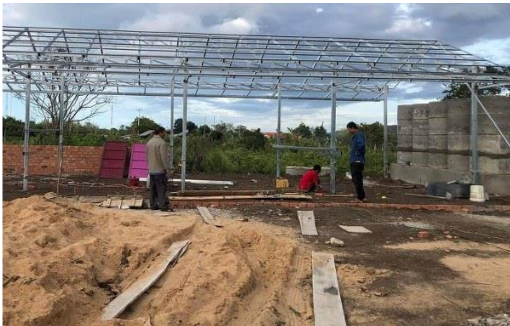
Dr. Samnang and his field supervisor visiting the progress of construction
