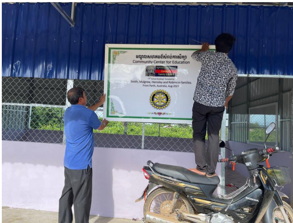
(The school completely built)
