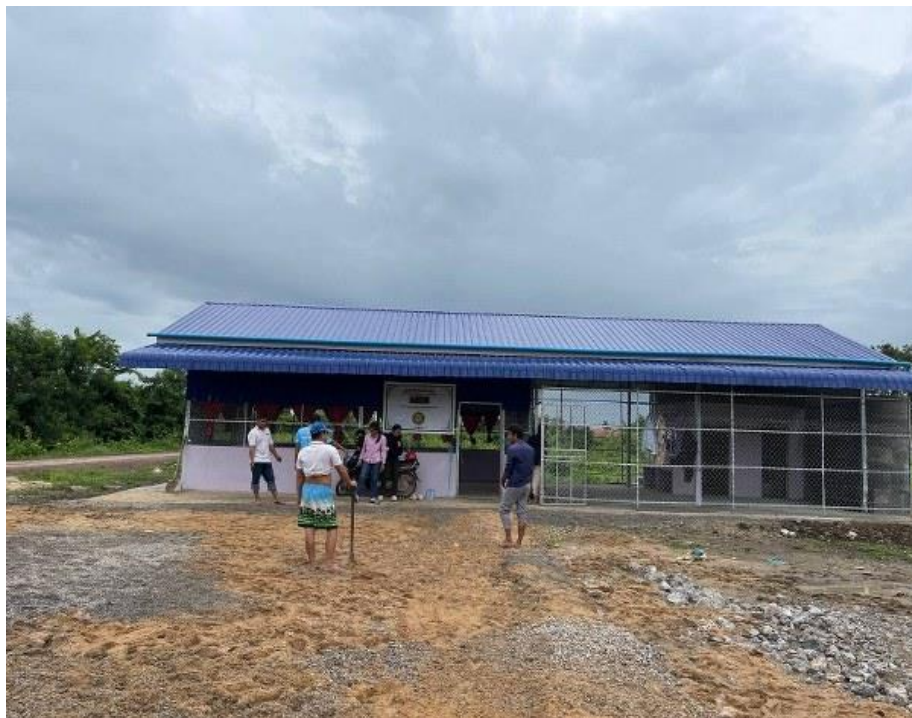
(The school completely built)
