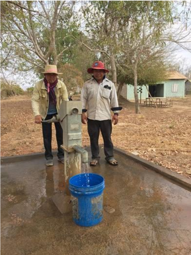
(Broken water well was fixed by CFS)
