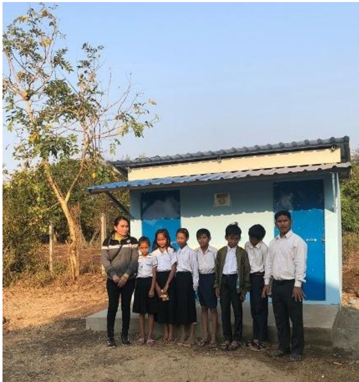
(School toilet completely built)
