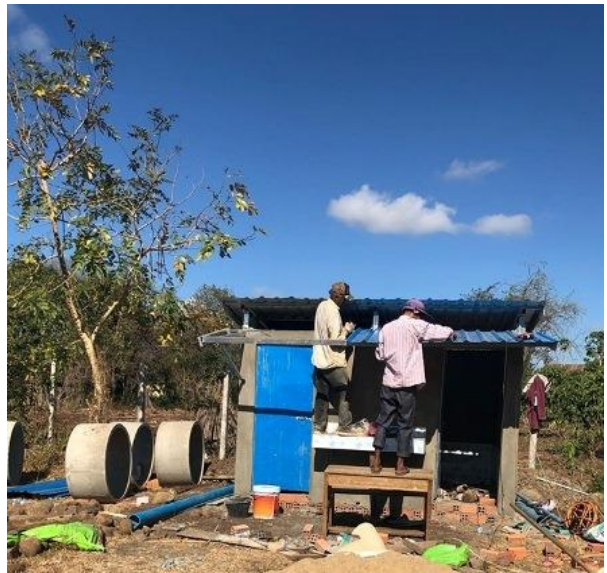
(School toilet is constructing)
