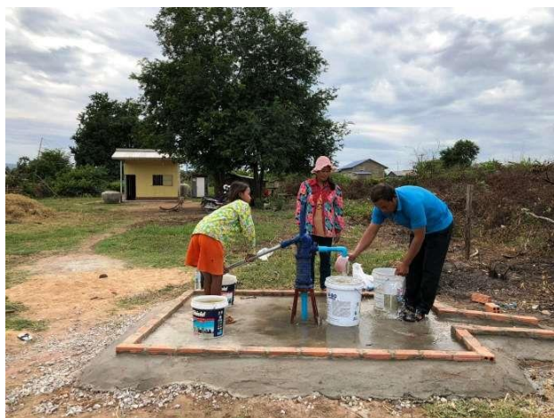
Communal bore well and pump supported by CFS
