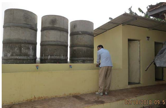
(Hand washing and school toilet built by CFS)
