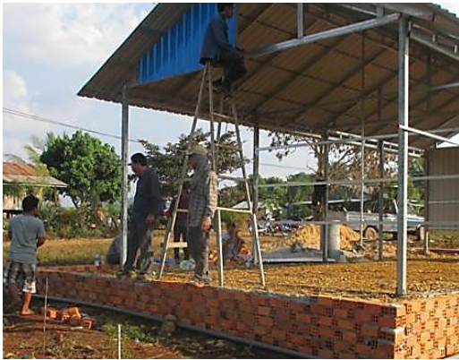
(Ongoing process of building)
