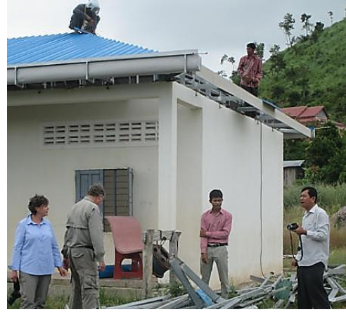
(Ongoing process of tin roof fixing)
