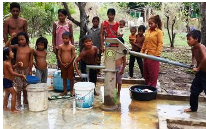
(Pump well fixed)
