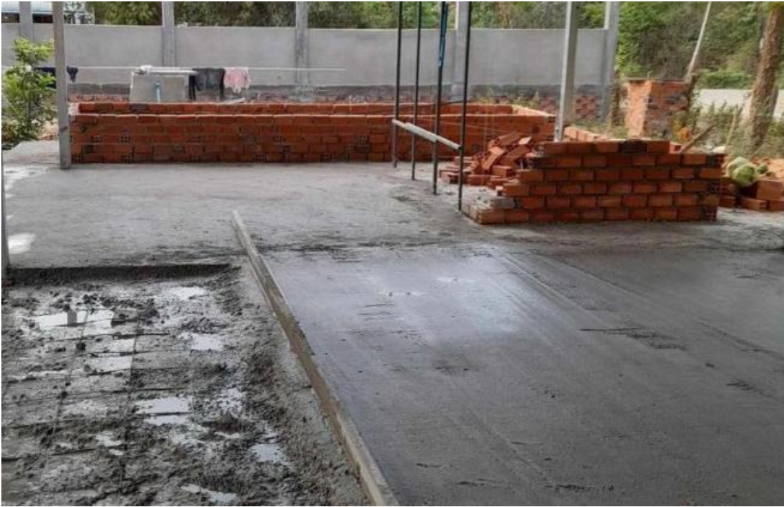
(The school construction started)
