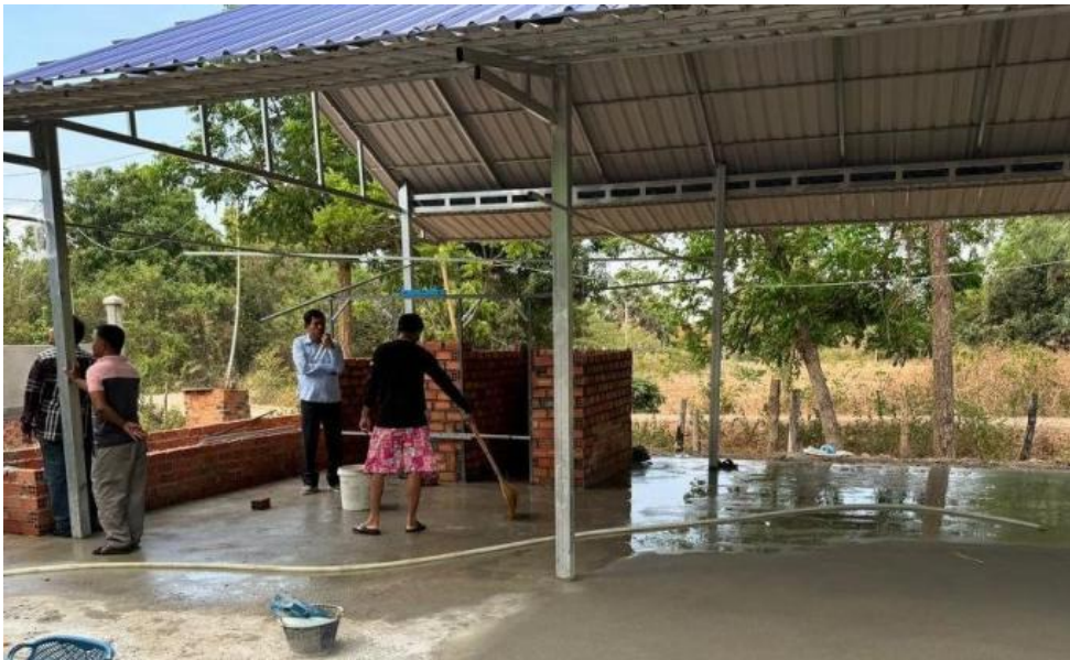
(Dr. Samnang visits construction progress)
