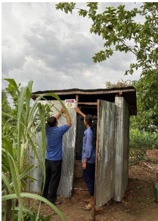
(The same place after completely latrine built)
