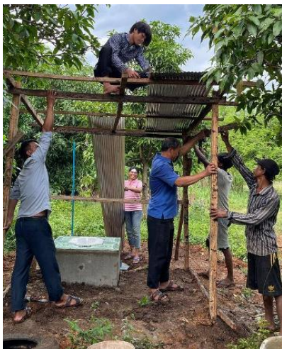
(They helped each other to build their latrine) (CFS-Photo)
