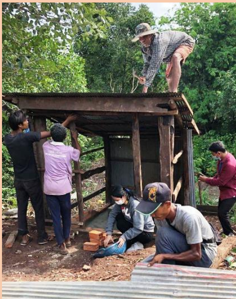
(They are helping each other to build their latrines)
