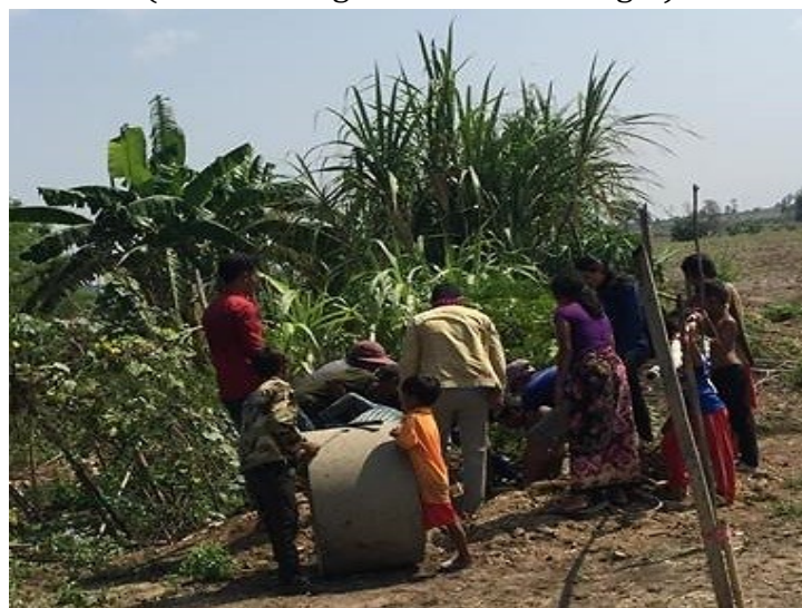
Helping together building their own toilet,
