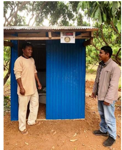
Latrine complete built
