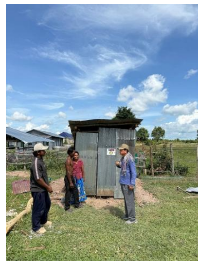
Latrine complete built
