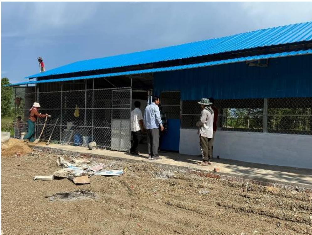
(Dr. Samnang and his field supervisor visiting the progress of construction)
