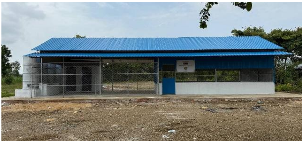
(Building is completed)
